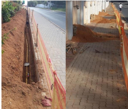
Trenches waiting for the arrival of Fiber Optic Cable
